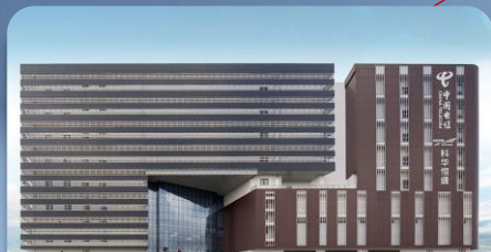
Guangzhou Desheng Data Center
