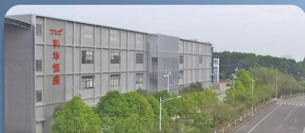
Guangzhou Keyun Data Center
