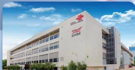
Guangzhou Qian Sheng Data Center
