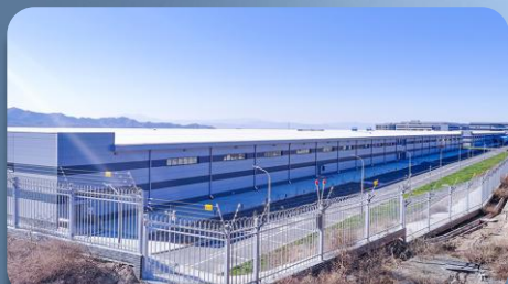
Zhangjiakou Tengzhi Data Center
