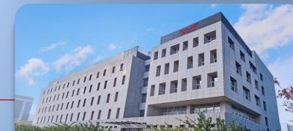
Beijing Zhongteng Data Center
